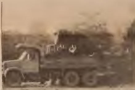
Hauling the earth out of the pond bed and over to other parts of the park that need filled in.
